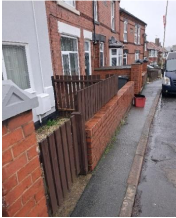
Image 15: Narrow pavement between 56 and 60 Hermitage Road, Whitwick
